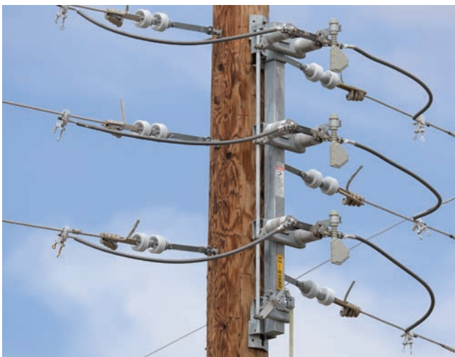
Figure 1. Tiered-outboard mounting configuration switch.
