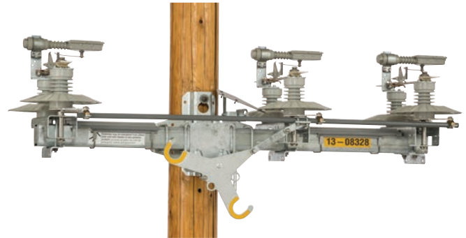
Figure 10. Phase-to-ground wildlife protection.
