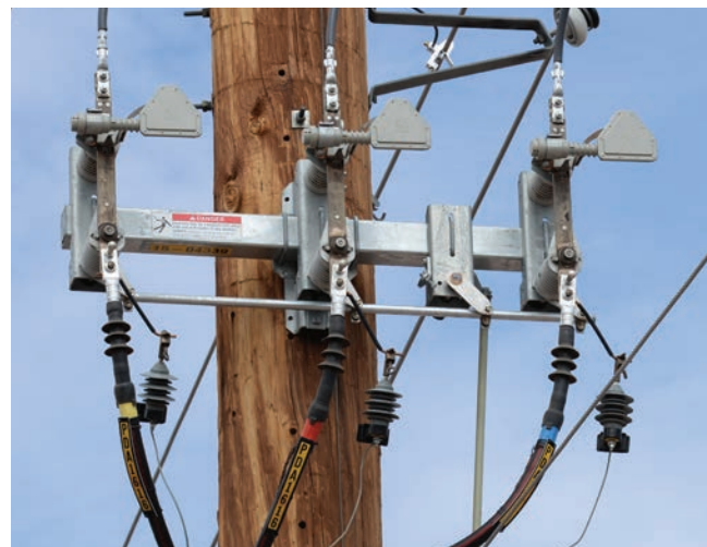
Figure 2. Vertical mounting configuration switch.
