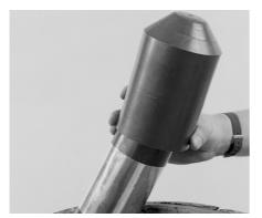
Wipe loose dirt from cable and slip end cap over the cable.
