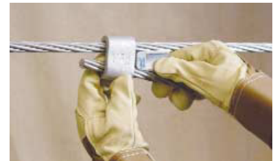
Place tap on conductor
