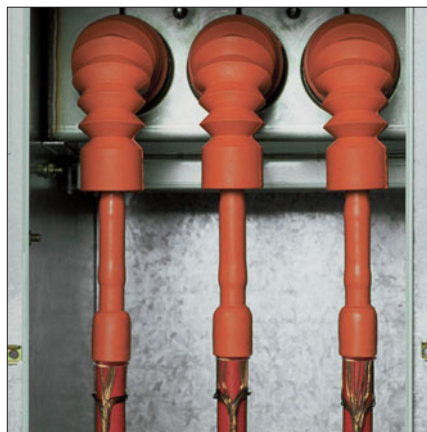
TFTI installed with Raychem bushing boot (RCAB)
