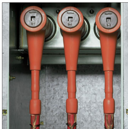
TFTI installed with Raychem insulated connection system (RICS)
